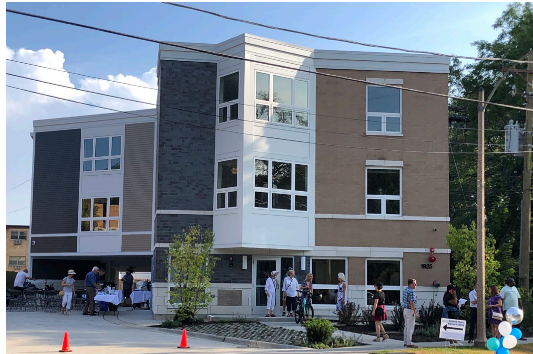
Cleland Place non-age-restricted affordable apartments, Wilmette Developer: HODC
