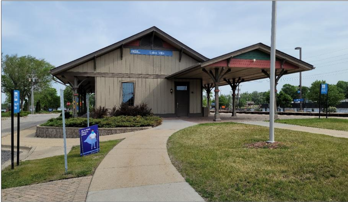
Figure 1.3: Lake Villa Metra Station
