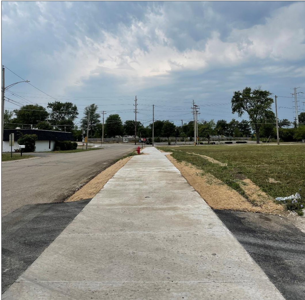
Figure 5.6 Installation of New Sidewalk on Cedar Avenue
