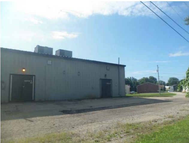
#15: View of the east adjoining alley and commercial strip mall beyond, facing southeast.
