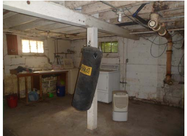
#8: View of the basement.
