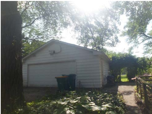
#3: View of the garage in the center of the property.
