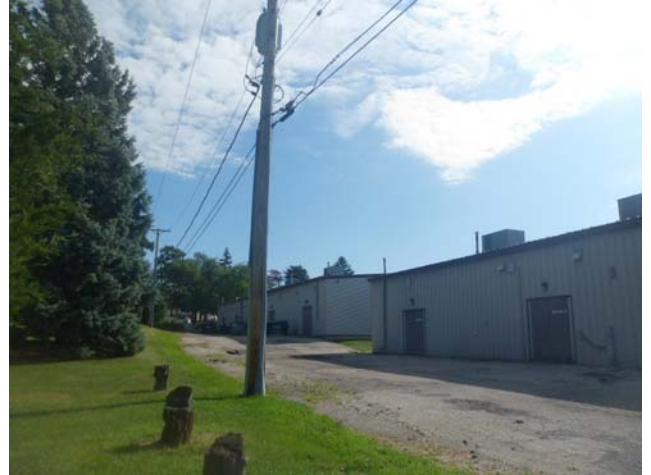
#14: View of facing northeast along the east adjoining alley.
