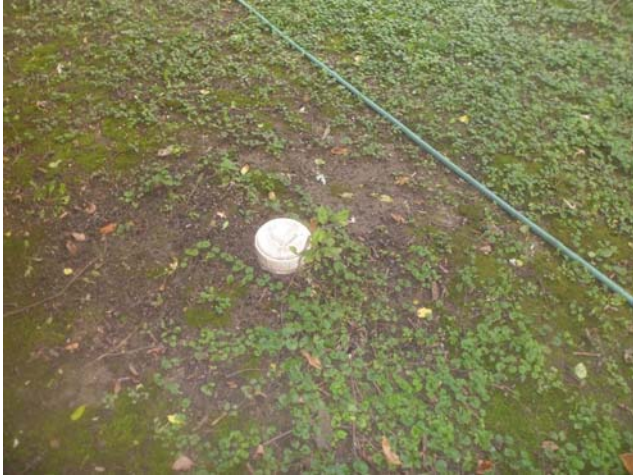
#19: View of the possible sump cleanout.
