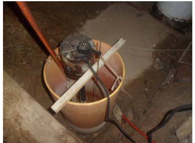
#18: View of the sump.
