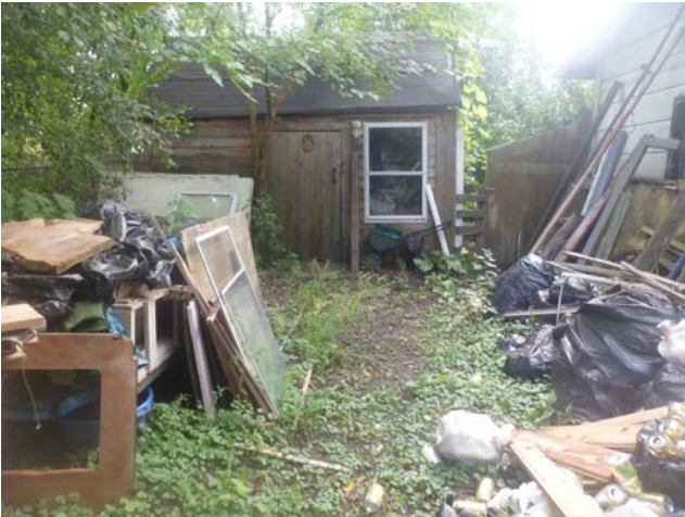
#9: View of the shed on the east side of the property.
