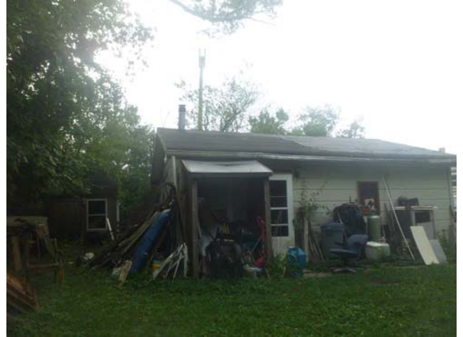
#8: View of the garage in the southeast corner of the property.
