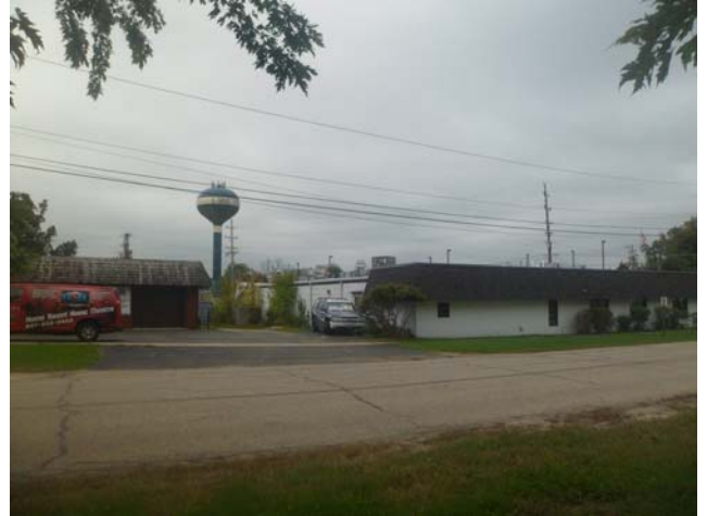
#20: View of the south adjoining Lake Avenue, beyond which is a vacant commercial structure (right) and HSH (left).
