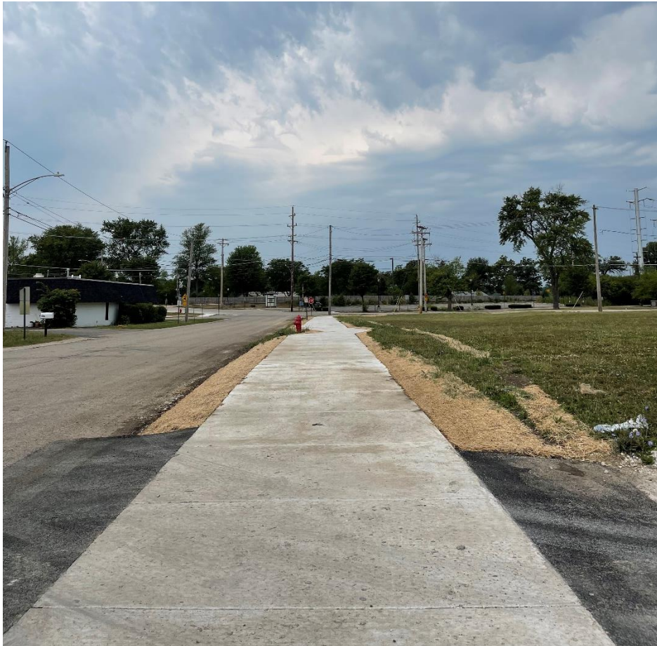
Figure 5.6 Installation of New Sidewalk on Cedar Avenue
